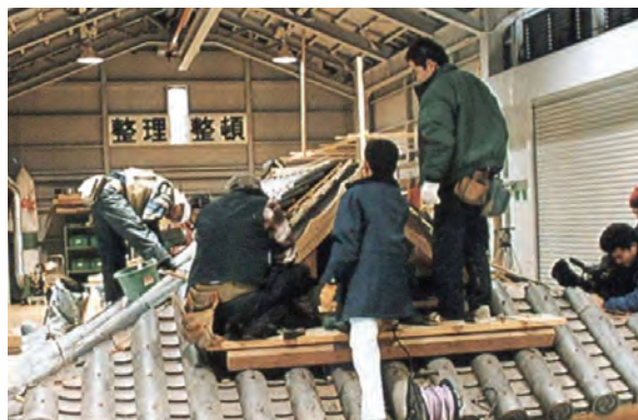
Practice work of tiling a roof
