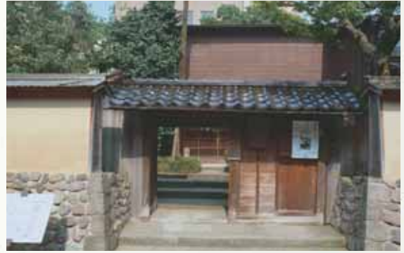
寺島蔵人邸跡 The Old Site of Mr. TERASHIMA KURANDO's House
